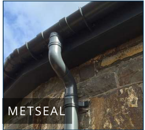
Fig 2. Powder Coated Anthracite Grey Cast Aluminium gutters along with some unusual angles (pictured) for which Rainclear arranged bespoke fabrication.
