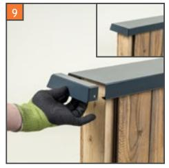
For stop-ends, apply a bead of silicone to the flange edges and push into position, wipe off any excess silicone. Affix a small rivet or selftapping screw to the back edge for additional security.
