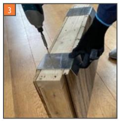
Once jointer bracket is in the correct position, screw in place using 4 screws per bracket, use No8 (4.0) countersunk screws or flat profile screw. Use the pre-drilled hole positions, or if these are not suitable drill additional holes.
