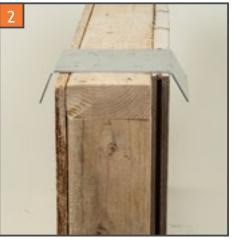
Position jointer bracket centrally over the wall, or if preferred align the front facing edge to the wall/cladding edge, leaving any overhang to the back. Brackets should be spaced at minimum 750mm centers (use a stringline to align the brackets)
