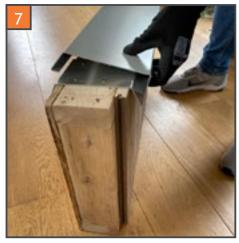
Using a rotation motion, push firmly down on the roof trim down until the sloping side clips into place. The bead of silicone should compress between the jointer bracket, wipe off an excess silicone.
