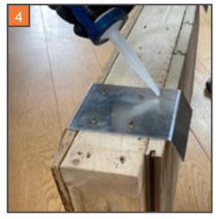
With jointer brackets in position, place one continuous bead (5mm) of silicone along the jointer inline with the screw heads. Use a Low-Modulus silicone.
