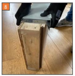
Ensure that the AluEdge capping is secure in place, and repeat steps 2-6 for the next length, maintain a 4mm expansion gap at every joint
