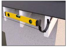
Create a fall of 1:600 to 1:350 (max) tying string from the first bracket (i.e. the highest) at one end of the gutter run to the last bracket (i.e. the lowest one - the one nearest the outlet and the downpipe) at the other end.
