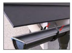
Fit the gutter lengths into the brackets and fold over the brackets' two 'tabs' to secure the gutter in place.
