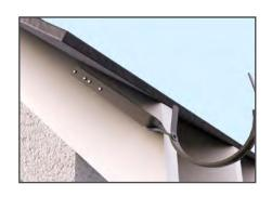
Fit the first bracket to the side of the first rafter on one outer edge of the roofline.
