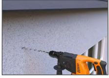
3. In the mortar between stones or bricks, make the hole with a chisel or old spike, or otherwise drill a hole to accommodate the spike.
