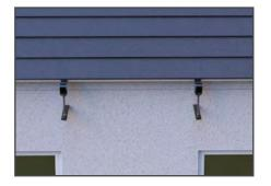
...tighten the nuts to set the bracket heights following the string guide now retied in the centre of the brackets.
