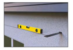
...creating a 'fall' of 2mm from the highest bracke the lowest one, nearest the outlet and the downpipe
