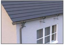
7. Insert the gutter lengths, and outlet into the brackets.
