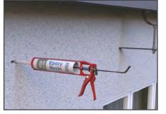
5. Apply cement or epoxy resin into the holes to secure all the spikes. A wooden wedge can help keep them in place, against the top of the hole, until they set.
