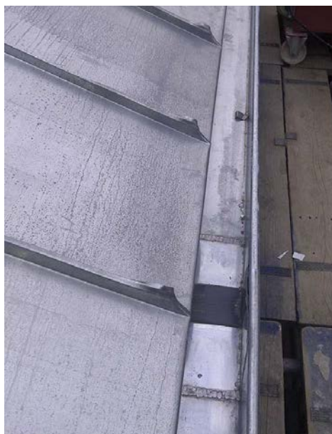
Expansion joint soldered to gutter
