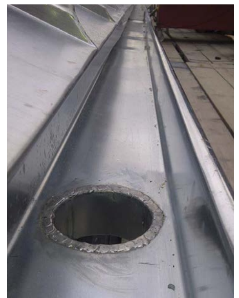
Downpipe outlet starter soldered to gutter
