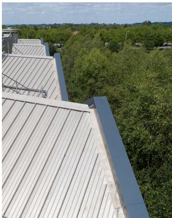
The unique trapezoidal plan and 'saw-tooth' roofline of the building had 7 gables, 14 valley, 1 corner, 2 end-caps. 16 unique angles needed to be measured and bespoke fabricated.
