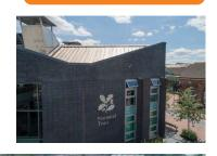
The unique trapezoidal plan and 'saw-tooth' roofline of the building had 7 gables, 14 valley, 1 corner, 2 end-caps. 16 unique angles needed to be measured and bespoke fabricated.
