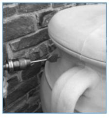
2. Fitting a Universal Fit Diverter with Filter or with Tap/Connection to the downpipe
