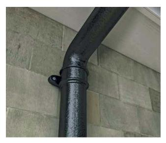
A range of traditional cast iron socketed round rainwater pipes in a choice of 3 pipe diameters and 2 pipe lengths. There is a comprehensive range of cast iron fittings, and traditional holderbat and earbelt fixings. Cast iron rainwater hopper heads are also available to suit.
