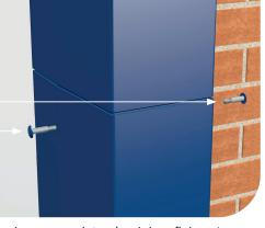
8. Secure the lengths, corners and bracket using appropriate aluminium fixings (use colour matched low profile self-tapping screw as shown). A minimum of two fixings are recommended on each joint and bracket.
