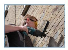
Alternatively, you may prefer to make a template. This is useful when fitting heavier canopies. Mark the template on the wall then drill your holes to receive the appropriate fixing. Once drilled, mark the frame using your template and drill the frame.
