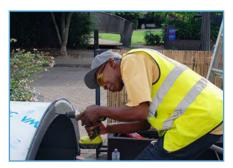
All of our canopy frames and brackets will need to be drilled by the installer prior to installation to locate the correct fixing points in the substrate.
