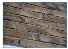
The installer should ensure that the substrate is sound and capable of supporting the appropriate fixings.
