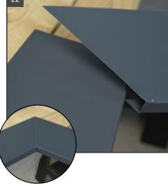
At the ridge, it is recommended to cut the profile so as to overlap the joint. The best way to achieve this is to run one gable through, then overlap with the opposite side. Once in position, fix the joint using 3.2 x 40mm nails
