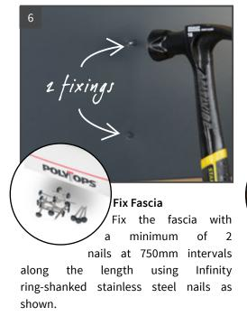
Note: All joints must be fixed through using 25mm ring-shanked stainless steel nail as shown above.
