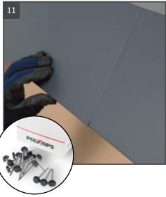
Fit the gable from bottom to top, this is important so that the overlap direction is weatherproof. Fix at 750mm centres using the larger fixing nail (3.2mm x 40mm).
