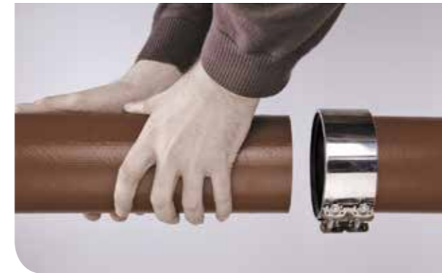
3. Ease the next pipe or fitting into the coupling as step 2.
