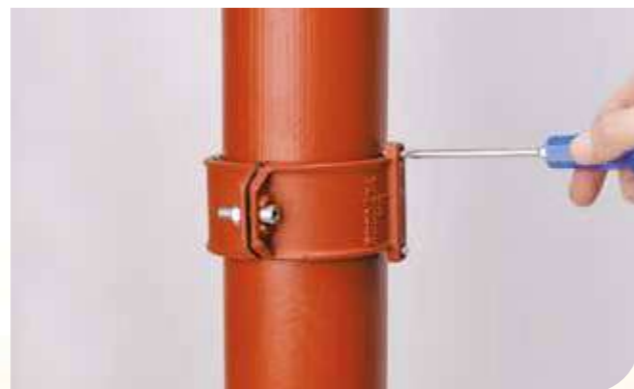
6. For electrical continuity, hand-tighten the electrical continuity screws on both sides. Ensure screws pierce external coating of pipe when tightened. (See page 55)
