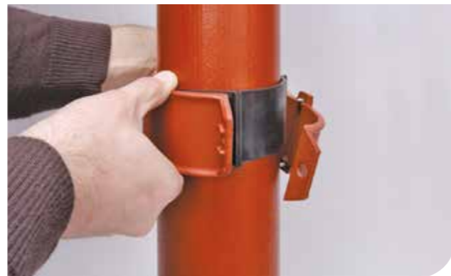
4. Loosely fit the coupling around the gasket, ensuring that the rubber lip sits into the corresponding locator in the coupling. The electrical continuity screws should be drawn back to fullest extent to avoid interference with the connecting pipe or fitting.
