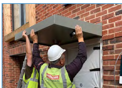
7. Slide assembled parts on fixed wall bracket (parts to be pushed tight against wall)
