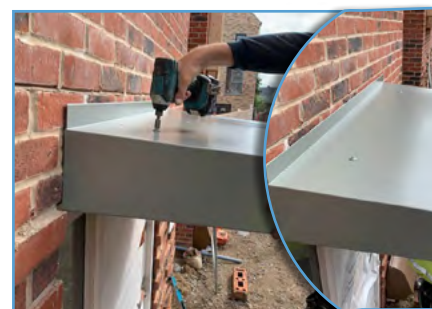
8. Secure parts by fixing through top to wall bracket using self-tapping screws with a rubber washer ( NOT INCLUDED ).
