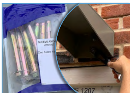
4. Install brackets with 100mm long M8 anchor bolts ( NOT INCLUDED – you will need to source these separately )
