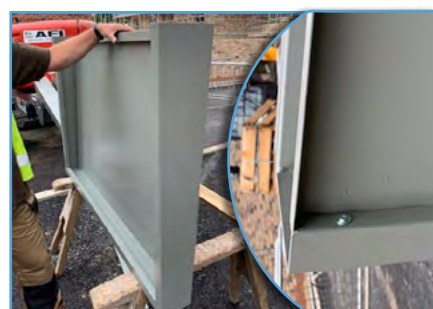
6. Assemble top section and soffit section with 4 self-tapping screws ( NOT INCLUDED ).
